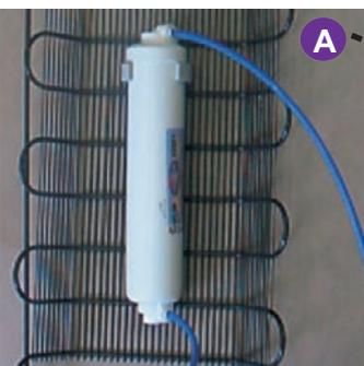
Block GAC (Granular Activated Carbon) filter
